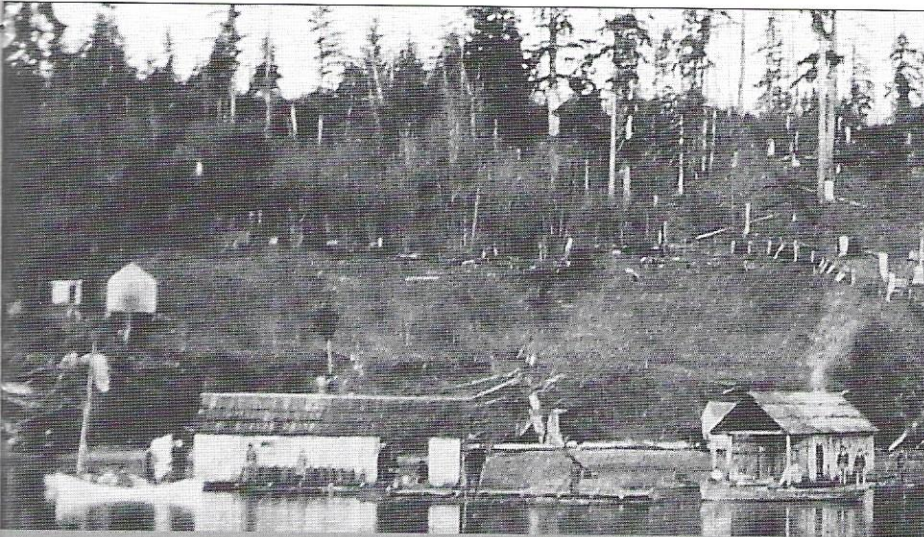
ABOVE: Katie Gale's home site and oyster beds. Her culling house and the associated float house can be seen here. RIGHT: Joseph Gale built a splendid home on Oyster Bay for his new wife Lillian around 1900. It was subsequently occupied by other families who worked the oyster beds.
